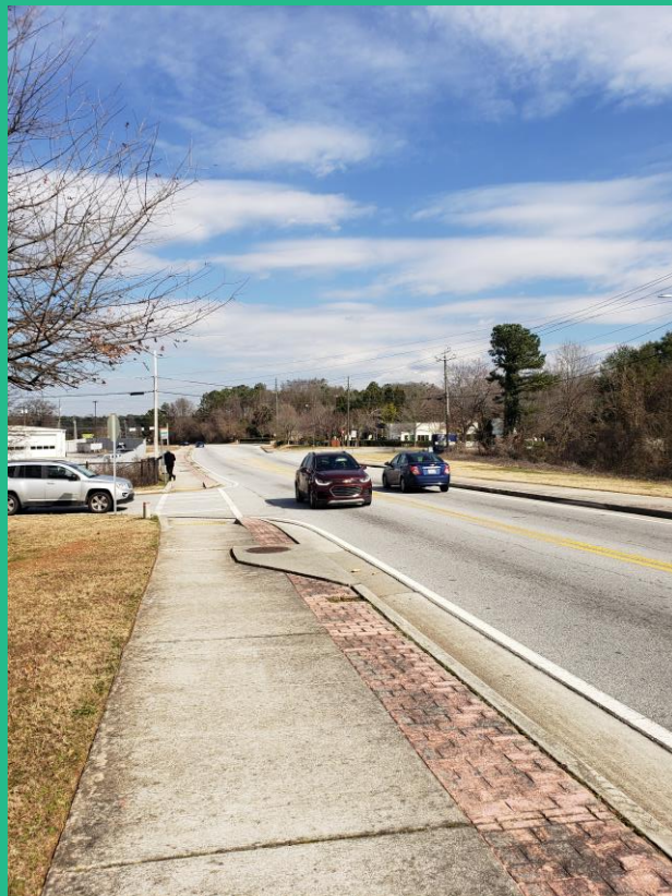
Figure 8: Cars passing down Montreal Road looking north towards Lawrenceville Hwy/US 29
