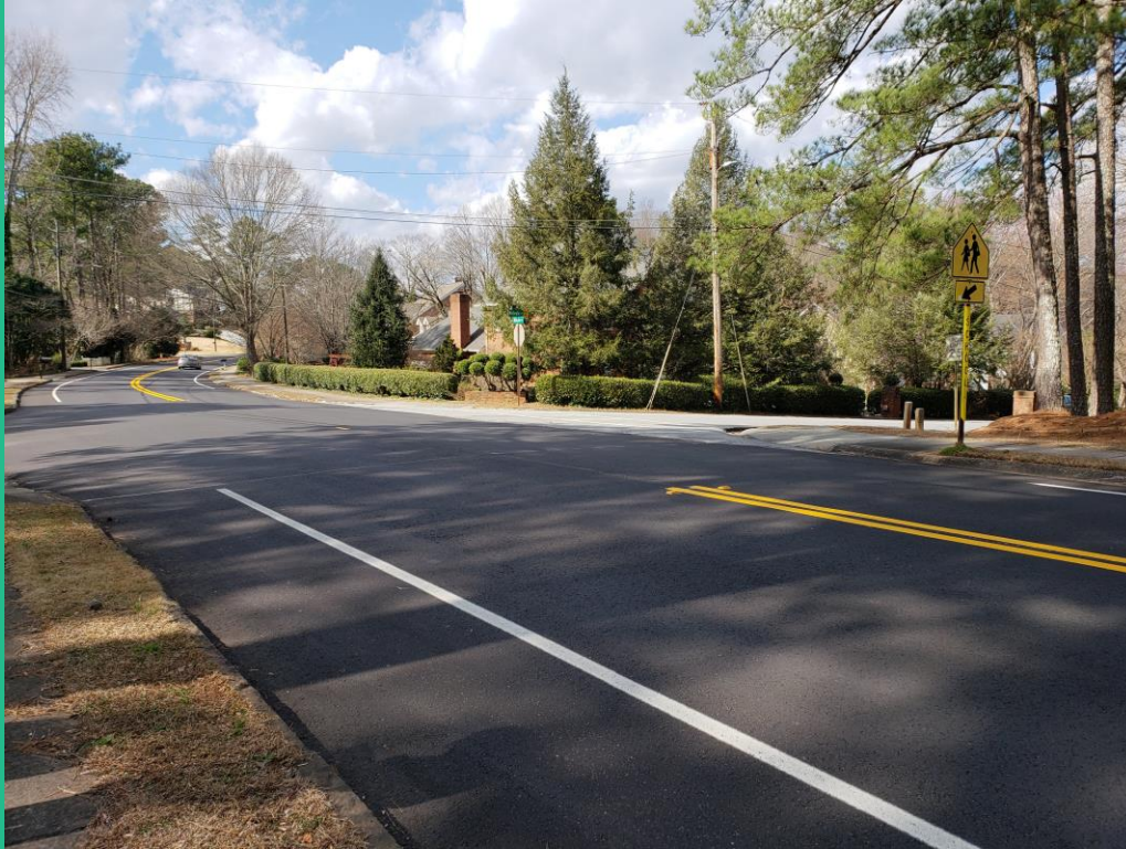
Figure 18: View of a crosswalk at the intersection with Midvale Court
