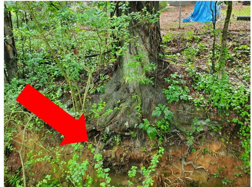
Bypass Channel - undercutting
