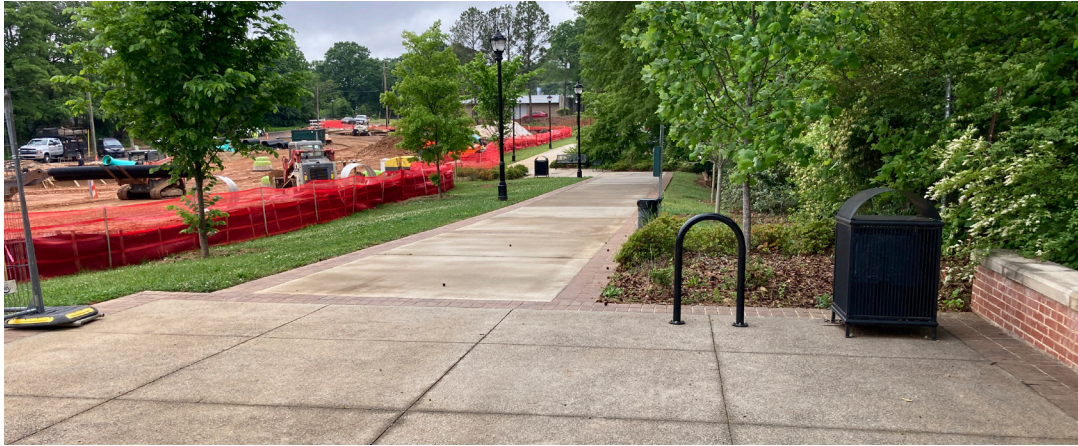
Construction of the new Tucker Town Green immediately adjacent to trail confluence plaza in downtown Tucker
